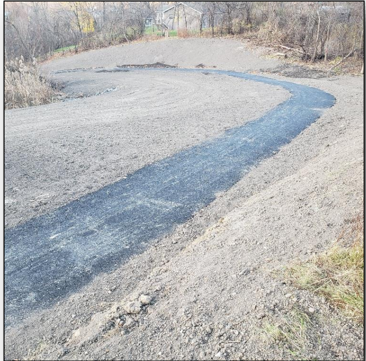
La Chute River Walking Trail under construction.
