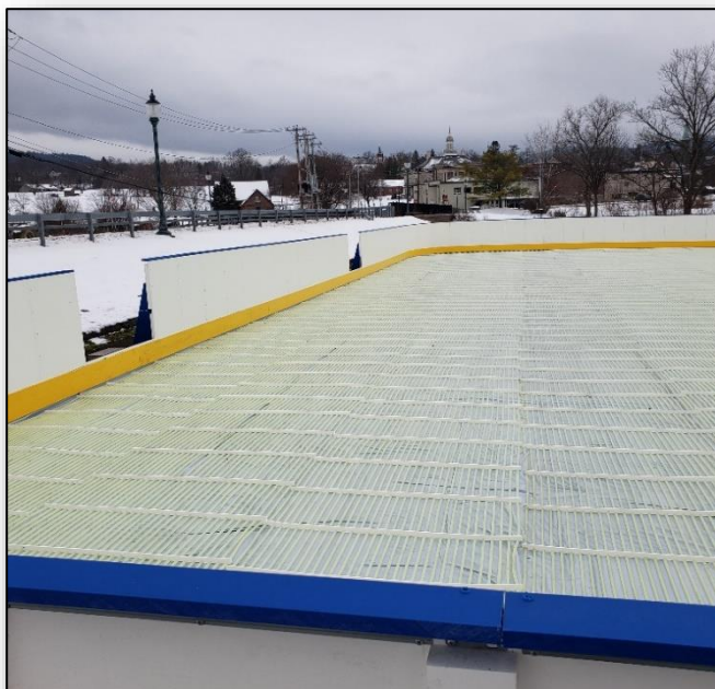
Rink installation completed.
