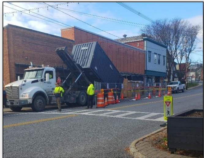
Work on 108 Montcalm Street begins.
