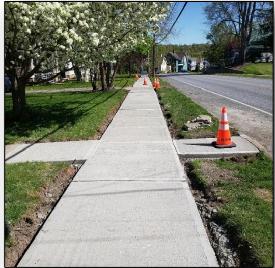
Sidewalk replacement on Lake George Avenue.
