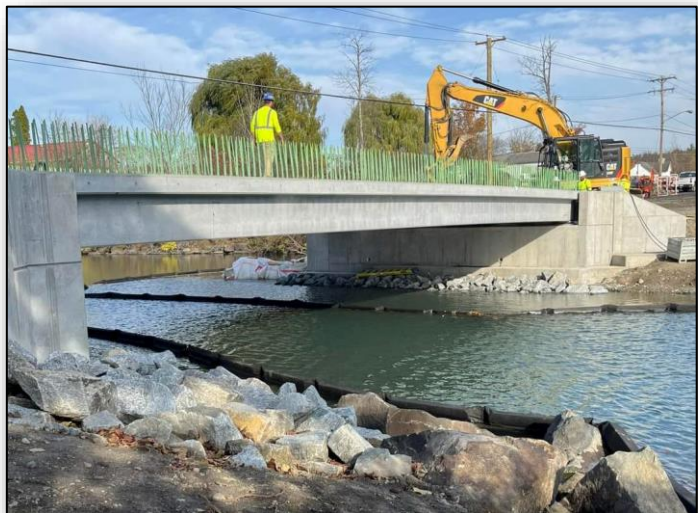
Alexandria bridge under construction.
