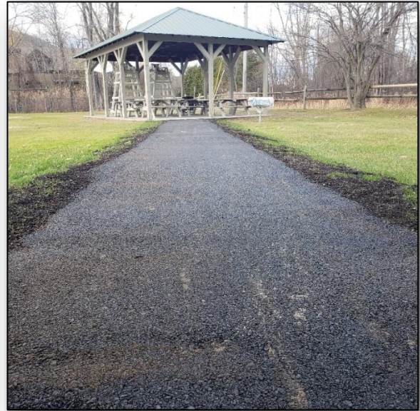
ADA Compliant Path at Beach
